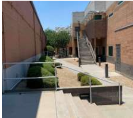
In between buildings adjacent to MA
